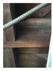
There are combustible materials that are within the 4" required clearance below the hearth extension. This presents a possible fire hazard. The masonry hearth extension can conduct heat that could allow the combustible materials to dry out and have a lowered ignition temperature over a period of time. The potential exists for these combustibles to ignite. Industry standard 2016 NFPA 211 11.3.1
