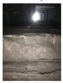
The smoke chamber walls are not parged smooth. This can cause a chimney to draft poorly. Lack of the parging material may also increase the risk of a structural fire and the risk of the byproducts of combustion migrating into the home. 2016 NFPA 211 11.2.1.13 IRC 2006 2111.S
