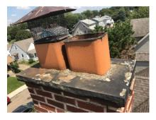
The stone crown of the chimney is attached to the tile with mortar. It will not likely be reusable when removed
