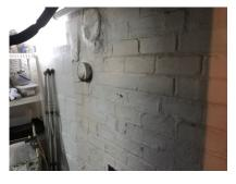
The clean out door is not in good repair and should be replaced 2016 NFPA 211 7.1.4.1
