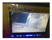
The tile is not sealed at the top of the smoke chamber
