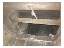
The firebox was blown out by the lightning strike. Bricks were laying on the grate after the strike
