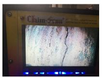
The lightning strike cased the surface of the tile to "pop" in a way that resembles flaking or spalling of the tile. This flue system is no longer capable of containing the byp
