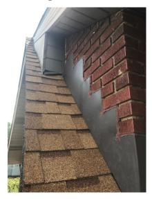
The flashing will need replaced after it is removed to allow for the chimney rebuild
