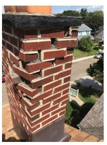
The bricks are no longer being held in place by the mortar. The chimney needs to be taken down to the lower roof and rebuilt
